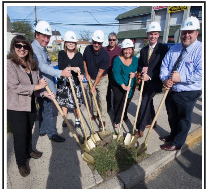
The Streetscape Phase I , ground-breaking took place on September 24th and construction began September 28th. (NJEDA Grant Award $1.5M)
